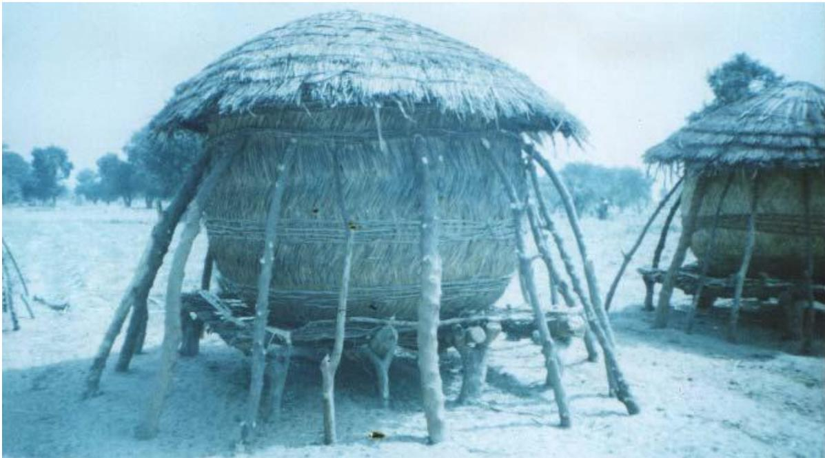
**Plate 4: Thatched Rhombus with tree stem columns, showing tree stem external support**
