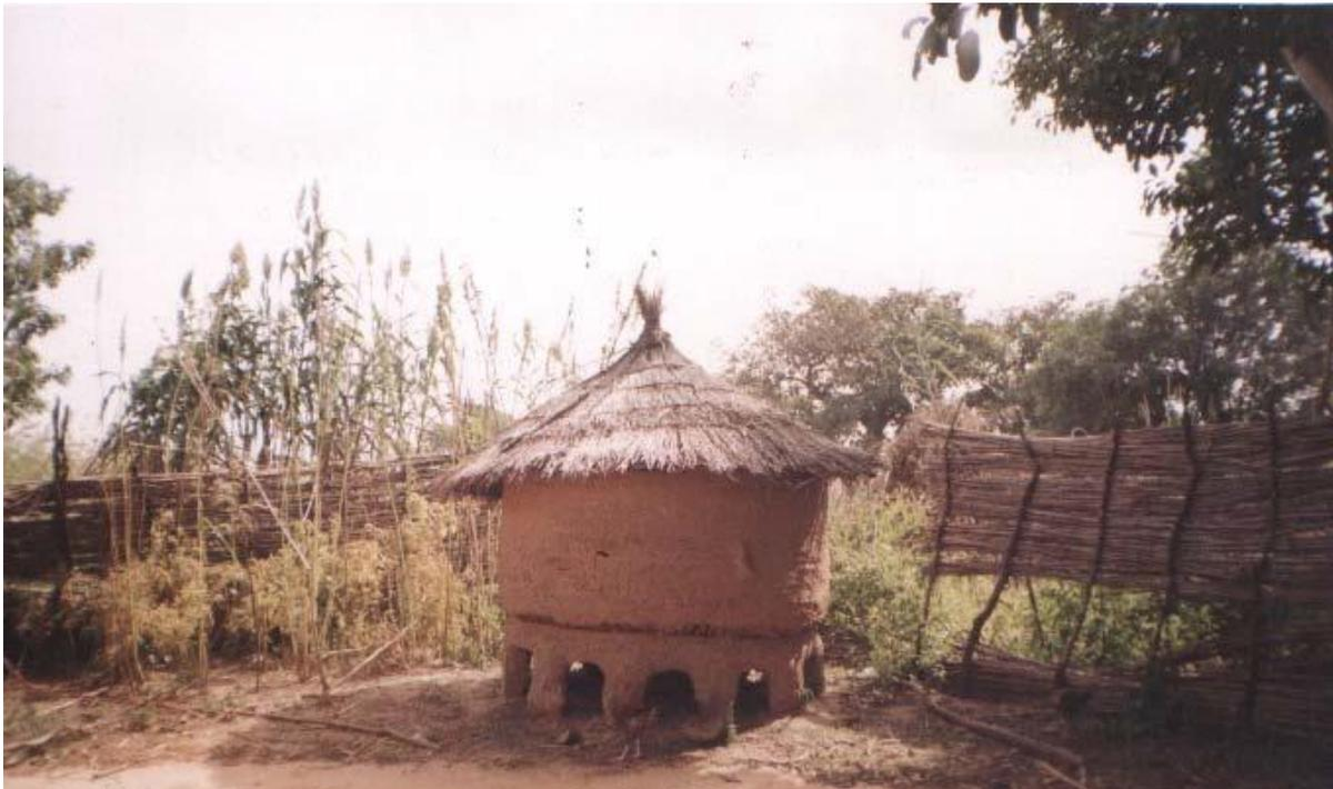
**Plate 3: Mud Rhombus with stone grillage foundation floor assembly and thatched roof**
