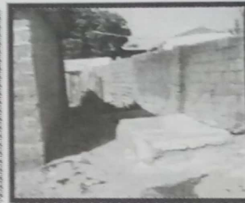
Fig. 9: Inaccessible Residential areas
