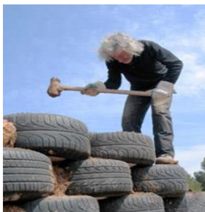
Plate 3: Conversion of discarded tyres in to an earthship. Source: Life.gaiam.com/article/garbage-warrior-turns-trash-green-built-houses
