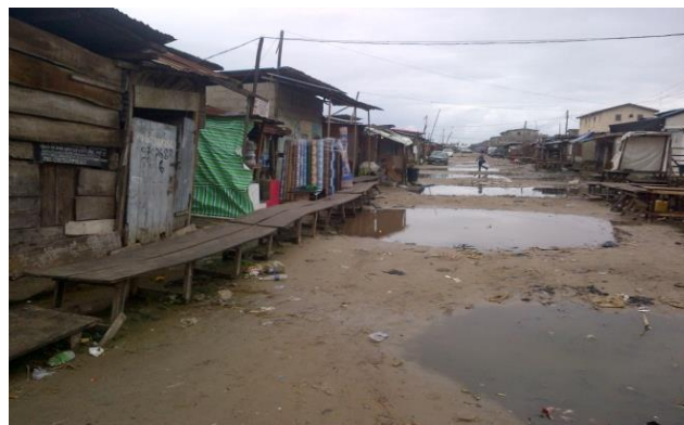
Plate 5.0: High congestion of poor building structures (shanties) on undeveloped estate land
