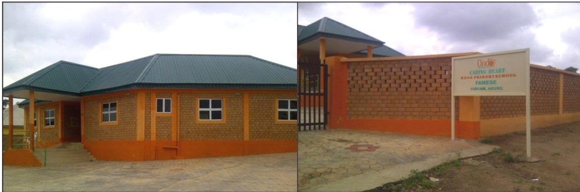
Figure 1: CSIEB used for the construction of a caring heart mega school, Famese, Isokan, Akure, Ondo state
