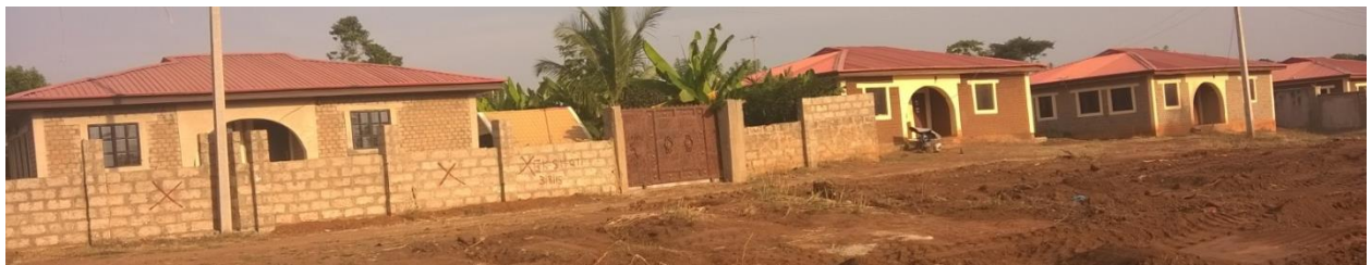
Fig. 2: Picture showing unapproved Fencing work under construction using Sandcrete blocks
