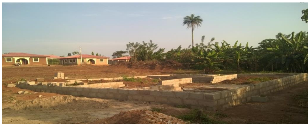
Fig. 5: Picture showing new construction still at Foundation stage
