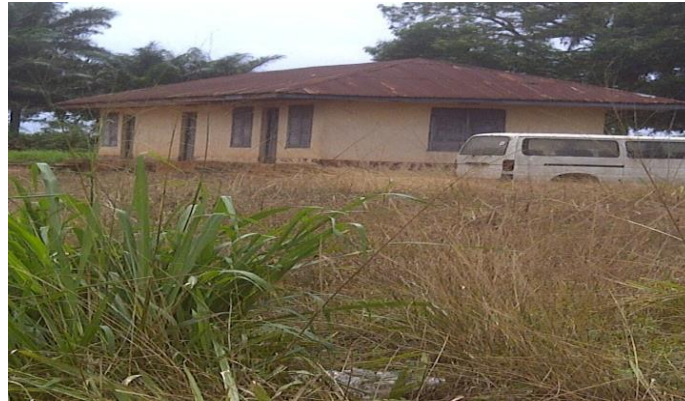
Figure 4: The Primary Health Centre in the community appears unused as it is overgrown with weeds
