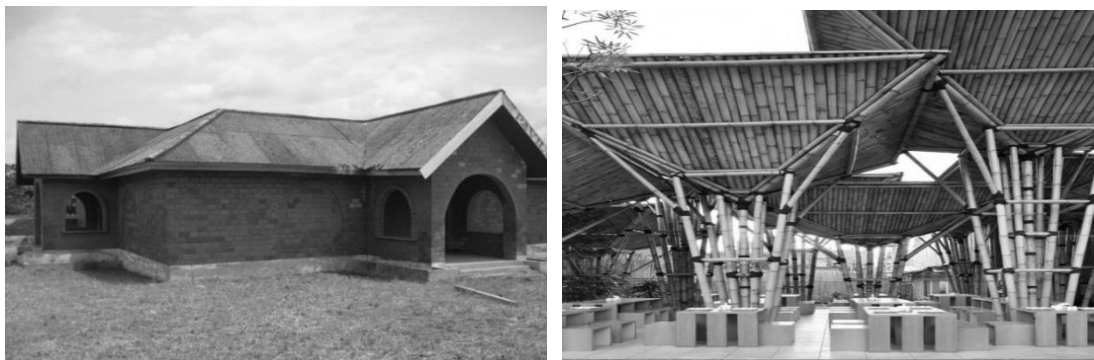
Figure 6: Showing a house made with laterite bricks and a recreation garden constructed with bamboo
