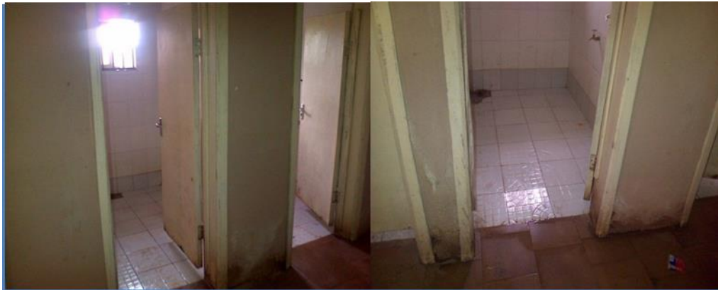
Plate 2: Bathroom facility in Adeniyi Hostel
