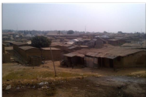
Plate 1: Unplanned structure on Paulossa
