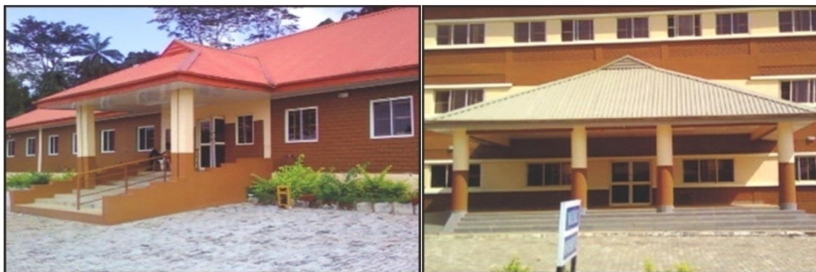
Figure 2: CSIEB used for construction of school clinic and hostel in Elizade University, Ilara-Mokin, Ondo state
