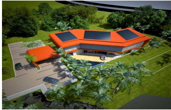
Figure 6 Idea House, Malaysia – Aerial view (Source: http://www.simedarbyproperty.com )
