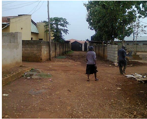
Figure 4: Abrupt Dead-end Road due to Poor Management of Infrastructure
