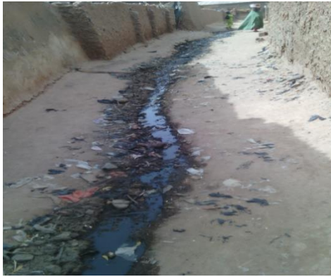
Plates 3 and 4: Hand-dug drains for Greywater in Palladan
