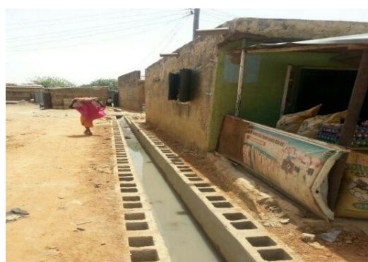
Plates 1 and 2: A stand-alone paved stormwater water drain along Kasuwan Mata street and a blocked drain in the study area
