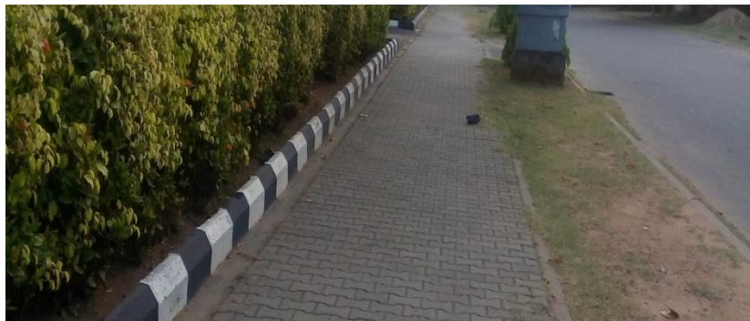
Fig. 6 Example of the use of permeable sidewalks and green lane in residential neighbourhood.
