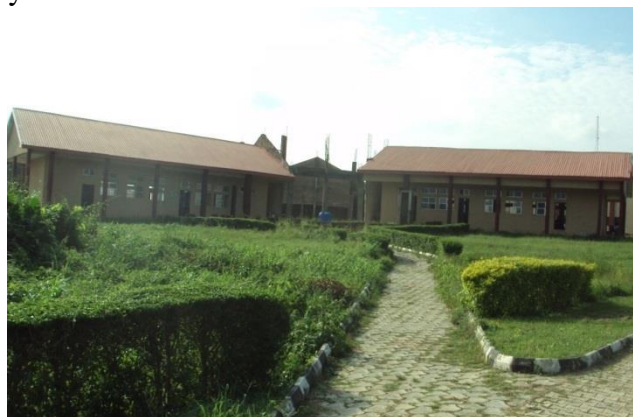
Fig. 2: Showing The Approach View Of The ‘3 In 1’ Lecture Hall With Verandas Serving As Horizontal Shading Devices.
