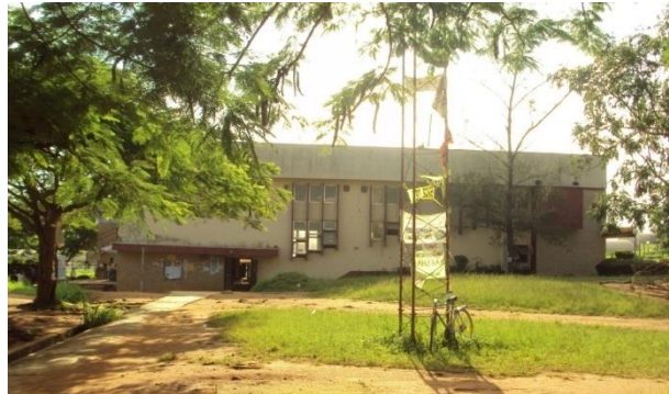
Fig. 1: A side view of the the Big LT showing the horizontal fins and the eave projection Source: Ojo (2013)
