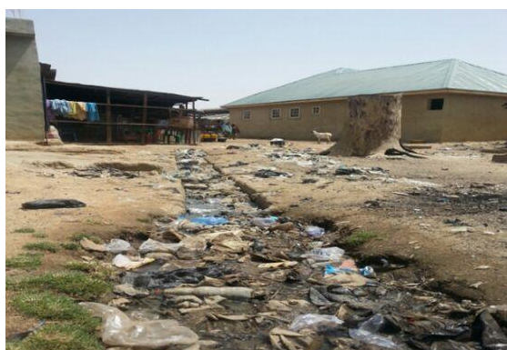
Plates 1 and 2: A stand-alone paved stormwater water drain along Kasuwan Mata street and a blocked drain in the study area
