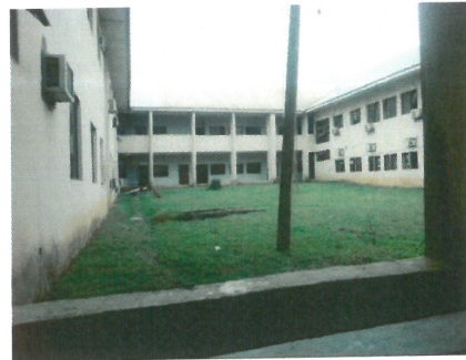
Plate vi: View of the courtyard Source: Author's field work (2017)
