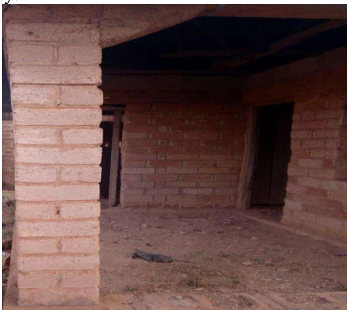
Figure 2: Earth brick column and walls
