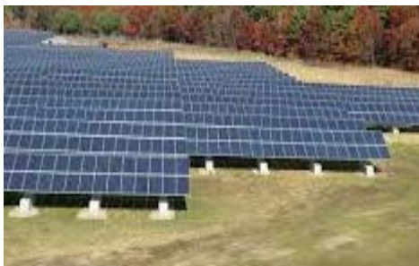
Fig. 12: Solar energy farm on category I reclaimed landfill
