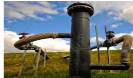
Fig. 6: Modern landfill gas well
