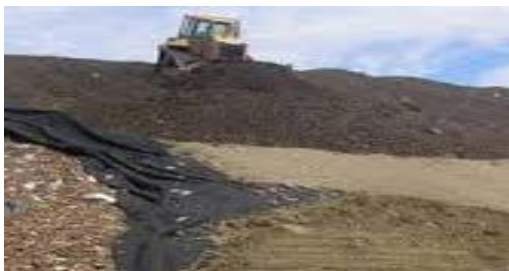
Fig. 16: Innovative biocovers spread as final landfill cover
