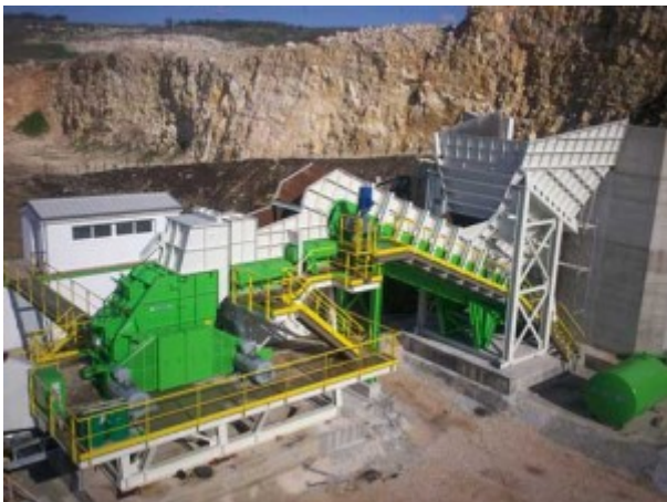
Figure 2: Bauxite mining and crushing site
