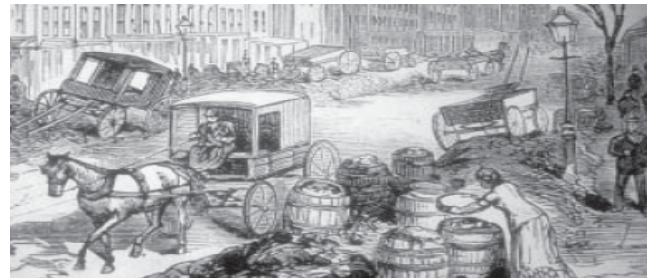
Fig. 1: Late 1800s city street side dumps (NSWMA, 2008)
