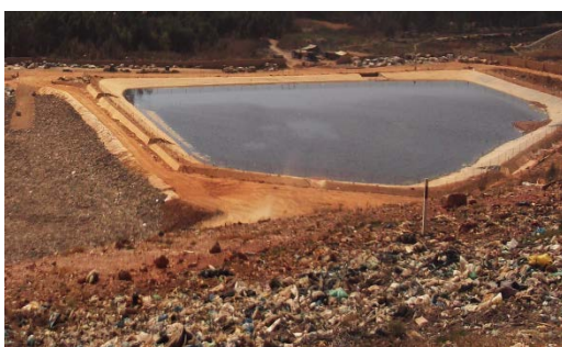
Fig. 10: Leachate basin in a landfill
