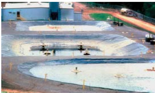
Fig. 9: Modern landfill leachate treatment facility (NSWMA, 2008)
