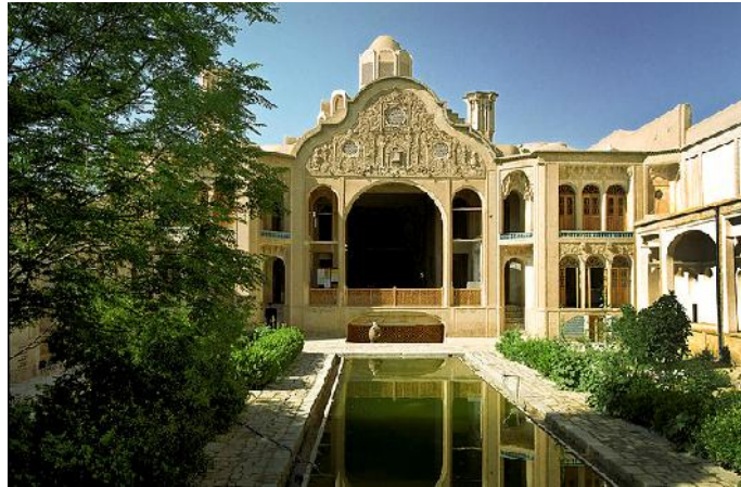
Figure 1: Boroujerdi-ha house in the Iranian city of Kashan
