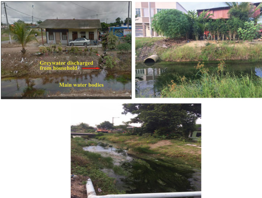
Fig. 2.1 Greywater discharge into the drain without any treatment. Photo was taken at 20/11/2016
