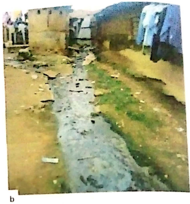
Plate 2(a&b): Discharge of leachate from unlined pit-latrine to the land surface in the study area
