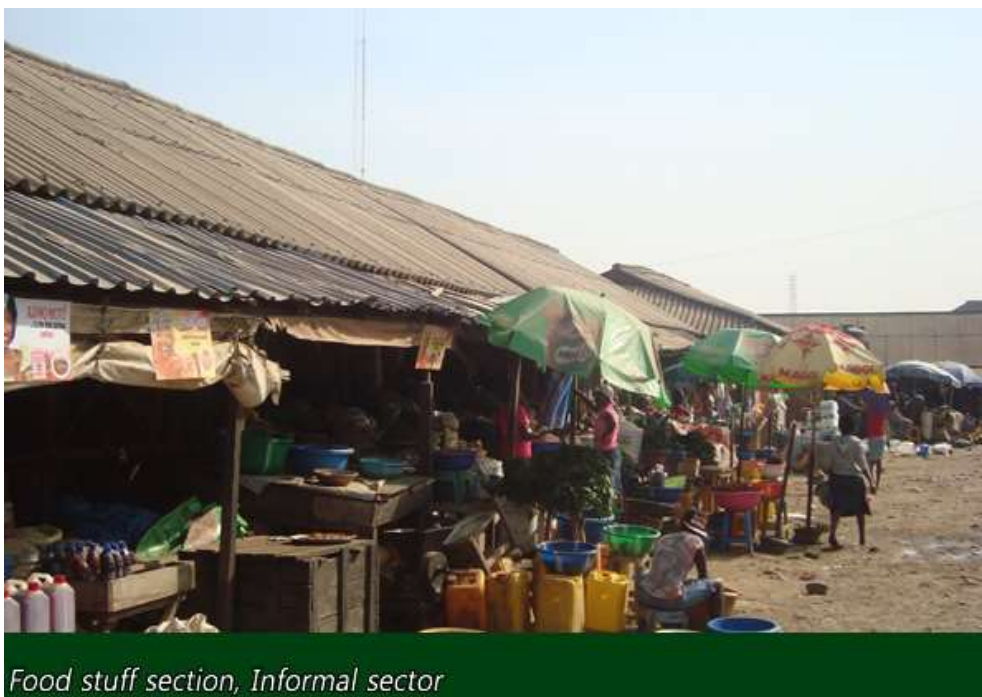
Plate XVIII: Over crowded nature of Kado market lock-up shops with non-fire resistant aluminium roofing sheets as sun shading device for corridor. Source: Abuja markets management limited, 2016 ( http://www.abujamarketsmanagement.com/kado-market/ ).
