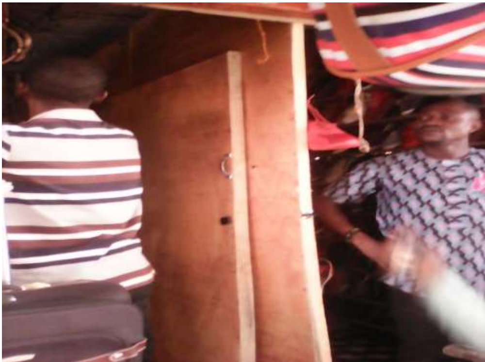
Plate XXI: Non-fire resistant wooden wall partition in a shoe shop in the central part of the formal section of Garki model market. Source: Field work (2017).
