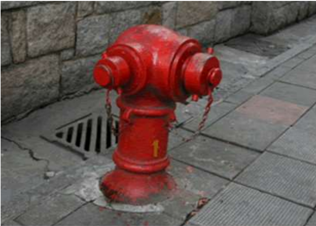
Plate VI: Street fire hydrant. Source: Department of fire services (special administrative region) of the Hong Kong government, 2003 ( http://www.hkfsd.gov.hk/eng/faq_safety.html ).
