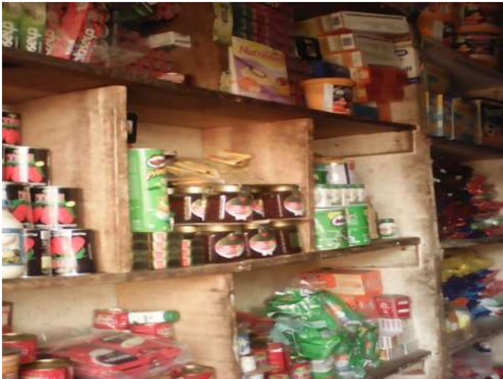
Plate XXII: Non-fire resistant wooden shelf in a provision shop in the central part of the formal section of Garki model market. Source: Field work (2017).
