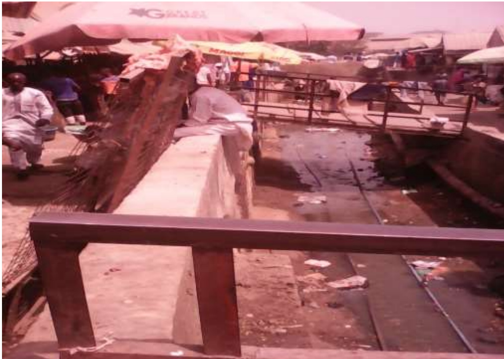
Plate XLIII: Canal in-between the formal and informal sections of Garki model market. Source: Field work (2017).
