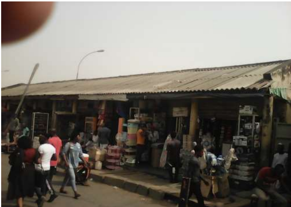
Plate LIV: Long gable roof without wall barriers against the spread of fires in the central part of Wuse market. Source: Field work (2017).
