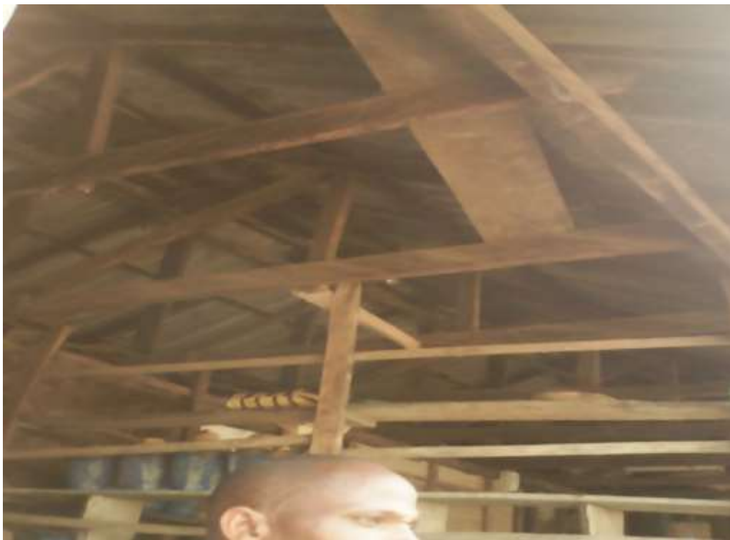
Plate LVIII: Non-fire resistant wooden structural members of the roof of an open stall in the central part of Kado market. Source: Field work (2017).
