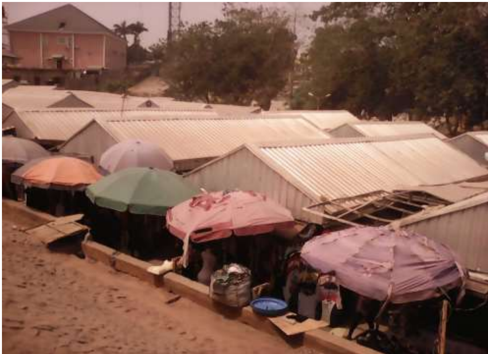
Plate LVII: Buildings with non-fire resistant aluminium roofing sheets in the eastern part of the informal section of Garki model market. Source: Field work (2017).
