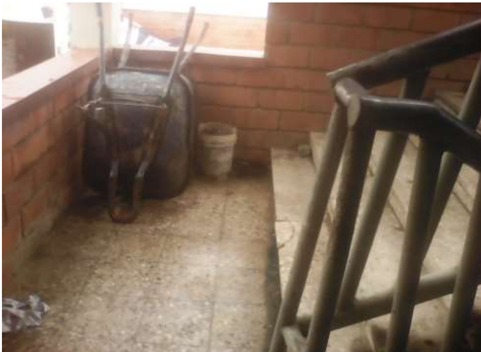
Plate XLVIII: Insufficient landing space in the northern part of the new section of Wuse market. Source: Field work (2017).
