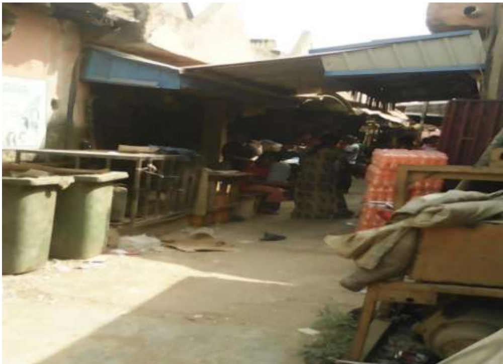
Plate XXVII: Corrugated aluminium roofing sheets that are attached to the buildings as a roof sun shading device around the cold room section in the eastern part of Kado market. Source: Field work (2017).
