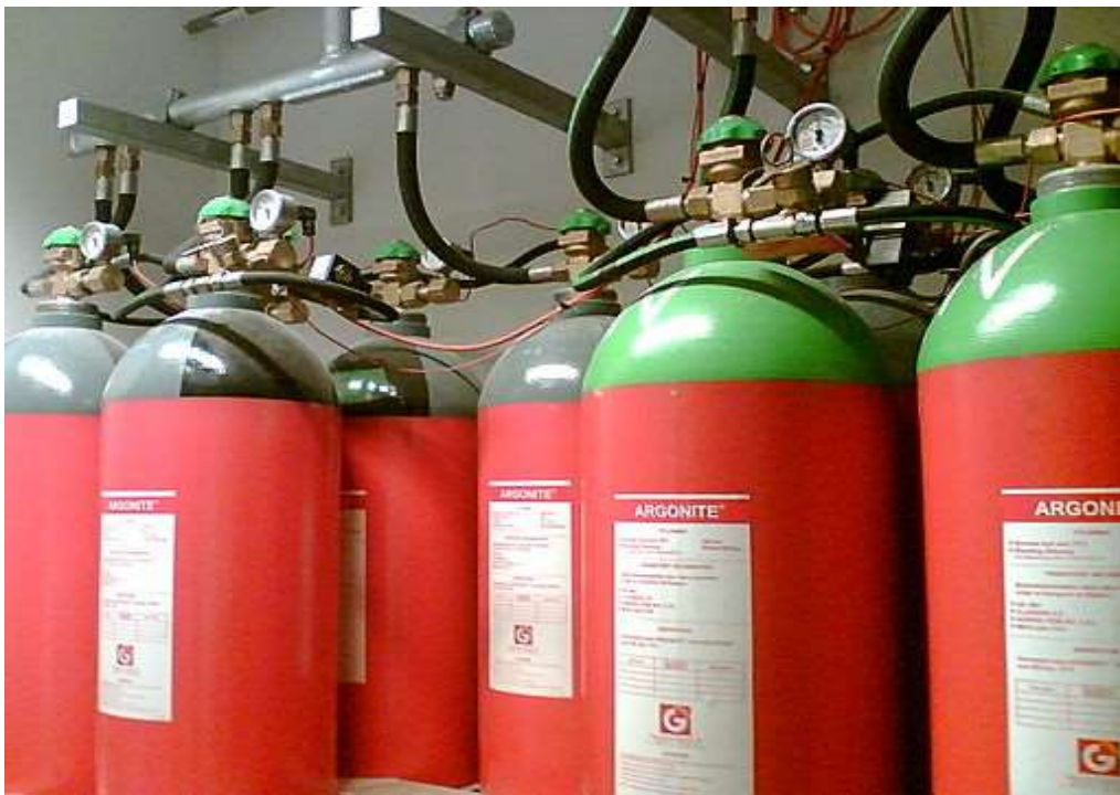
Plate V: Automatic fire suppression equipment. Source: Word press, 2013 ( https://bestfiresuppressionsystems.wordpress.com/ ).
