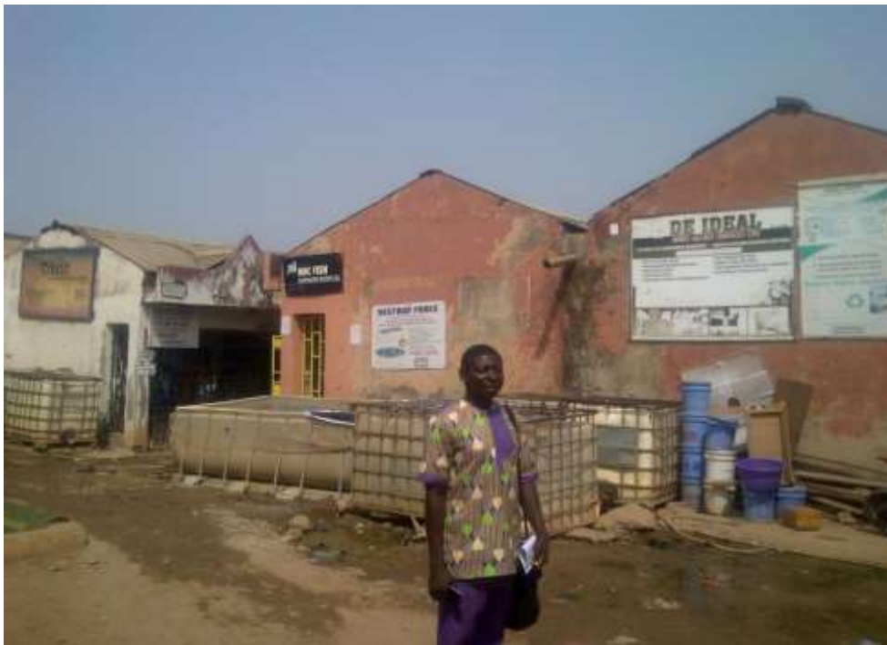
Plate XLV: Joint buildings in the eastern part of Kado market Source: Field work (2017).
