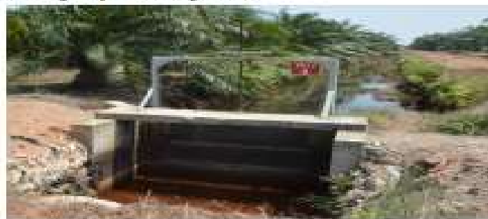
Figure 1. Installed Weir within the Peatland to Control Water Level.
