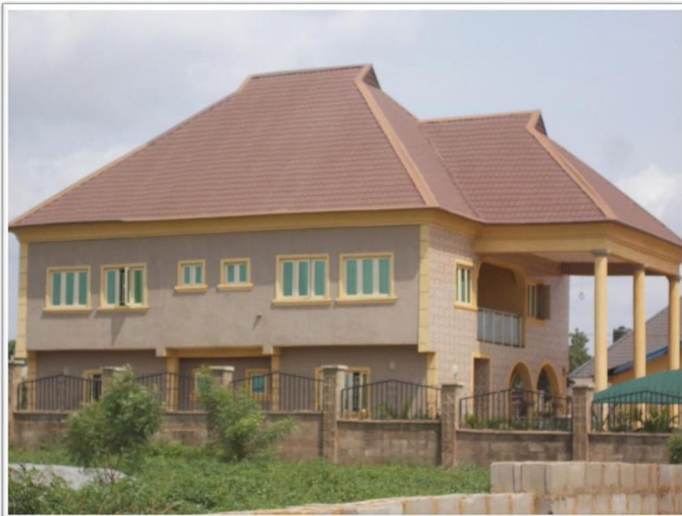
Plate II: Good wall of a building at Evergreen housing estates
