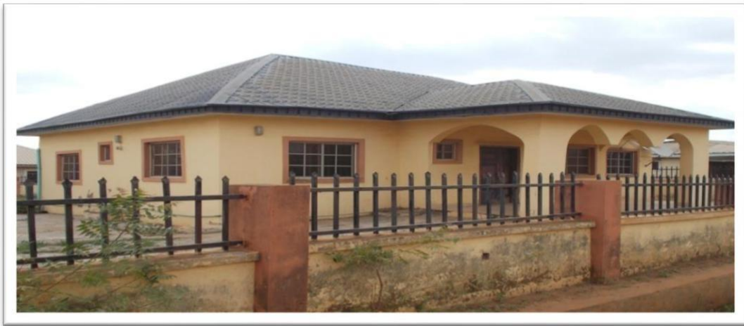
Plate VI: A building showing windows intact at Evergreen estate
