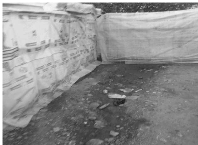
Figure 6. Drainage System at Kuchigoro Camp
