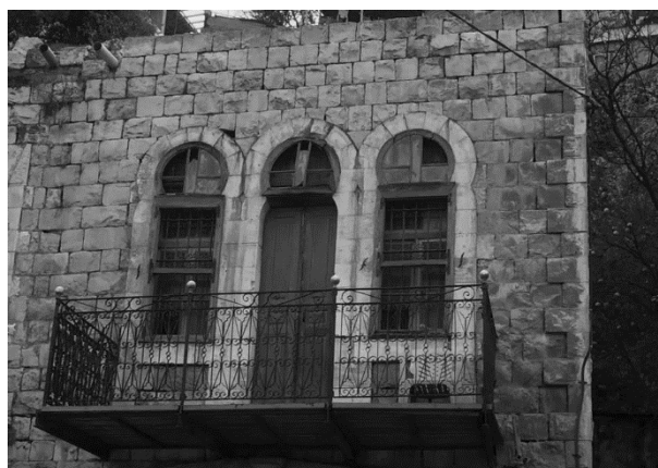
Figure 6. The windows are now enlarged, and the terrace system has emerged
