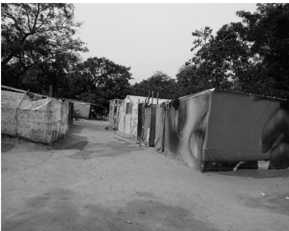
Figure 9. Shelter Condition at Durumi Camp
