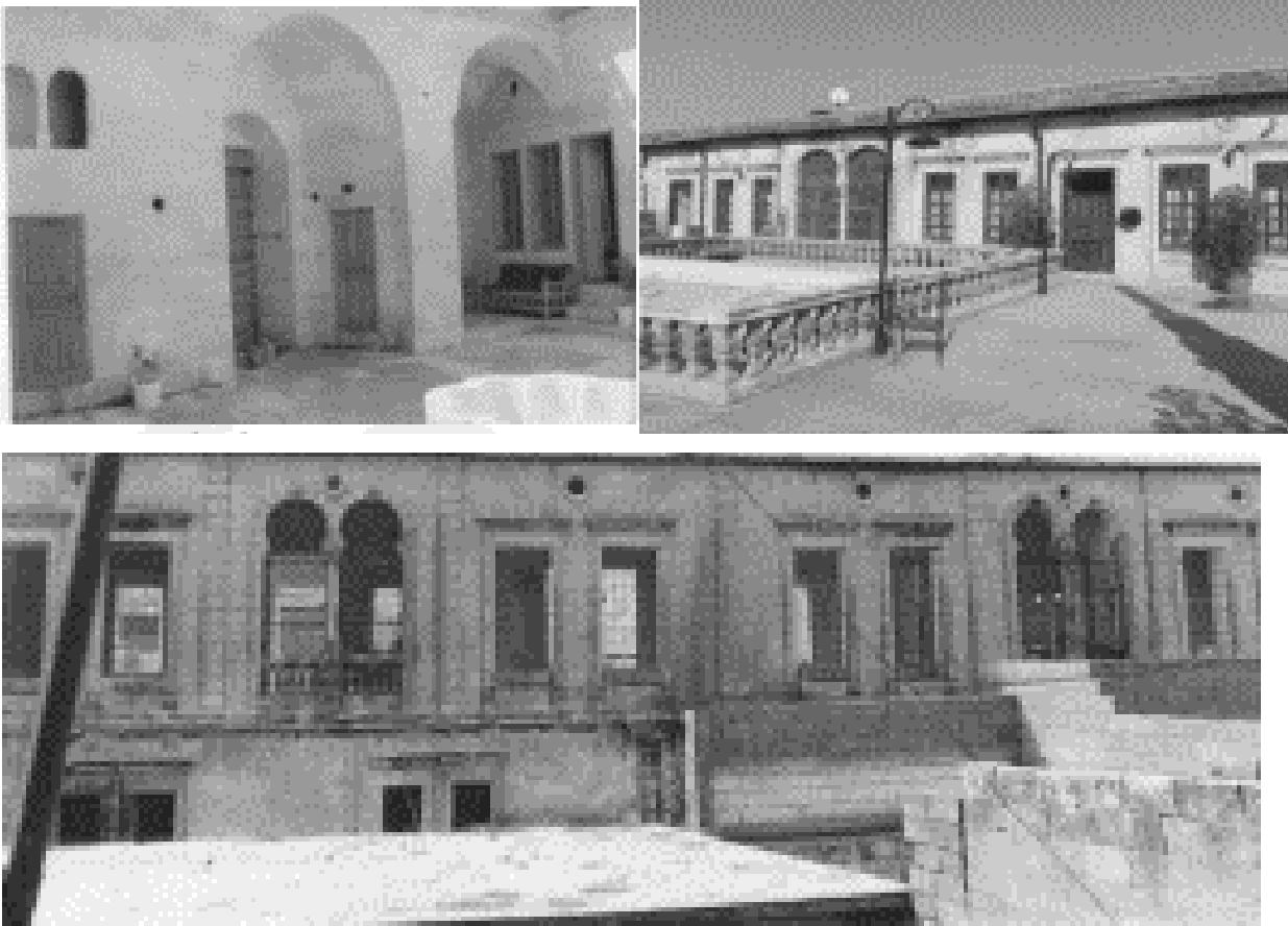
Figure 15. State Guest House, Courtyard Photo (left), Terrace Photo (middle), North Façade (right) (Kürkçüoğlu C., 1995)
