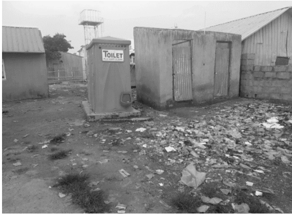
Figure 7. Toilet Facility at Kuchigoro Camp
