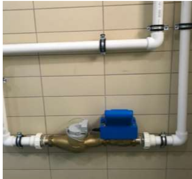
Figure 5. Installation of a smart meter for post meter leakage detection
