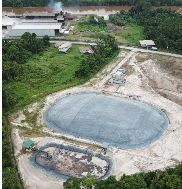
Fig. 1: Development of an integrated sago waste recovery, treatment and utilization demonstration plant in Mukah, Sarawak
