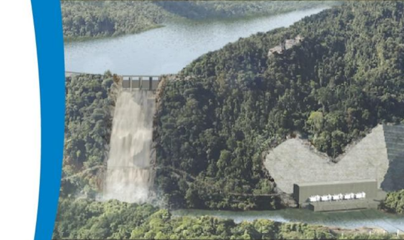
1,285MW Baleh Hydroelectric Project Target Commercial Operation Date: 2027
