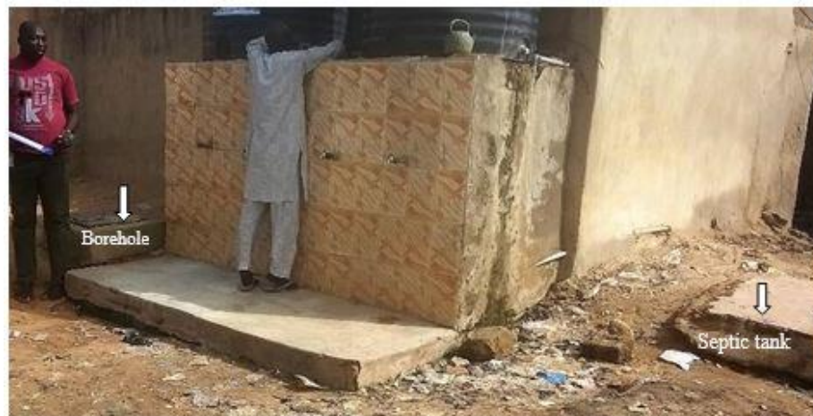
Figure 6: Public water supply in Bida with borehole and septic tank in close proximity
