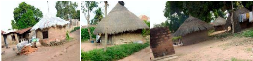
Plate 1: Showing unauthorised building subdivision, building materials and building conditions in Gaadi area, Makurdi, Benue State (Source: Researchers’ field survey, 2021)
