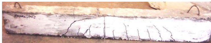
Plate III: Crack pattern for flexural failure of beam
