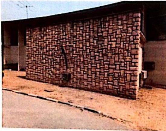
d). stone rubble decoration at national museum, Lagos
