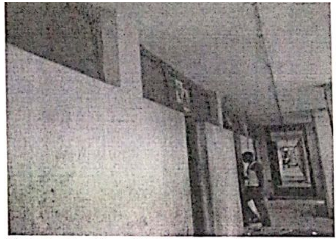
Plate 5: Corridor of Male Hostel Bedroom Of Male Hostel Niger State Polytechnic Zungeru. Source: Field Work (2015)
