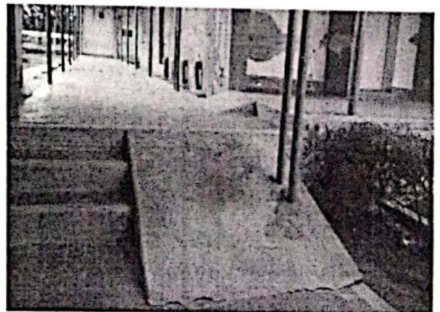
Plate3.Ramp at the School of Science and Science Tech (Too
