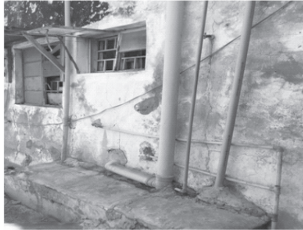
Plate 4.2: State of the facility and mechanical works
