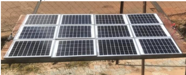
Figure 3: Experimental Setup for Unshaded Condition.
