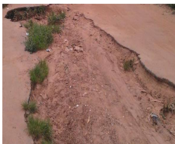
Plate 10: Failed road sections along Minna – Tegina and Tegina - Makera federal road
