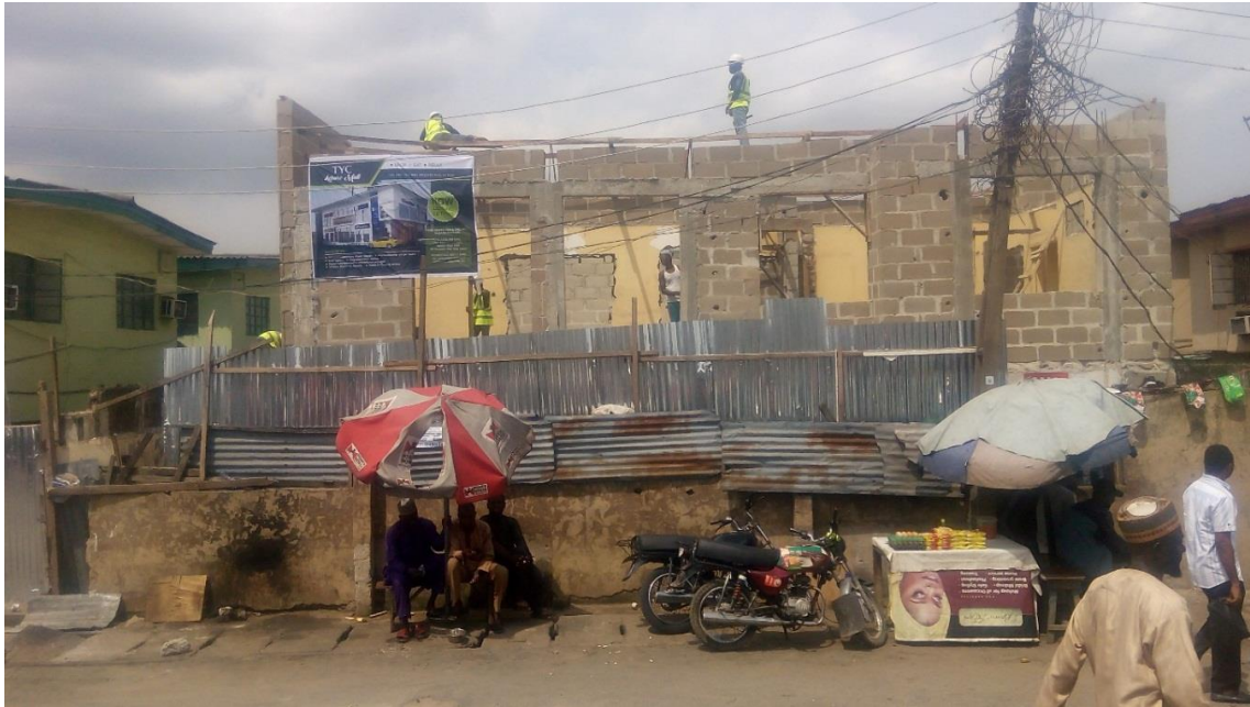
Plate IV: On-going alteration/ conversion exercise in Ikeja
