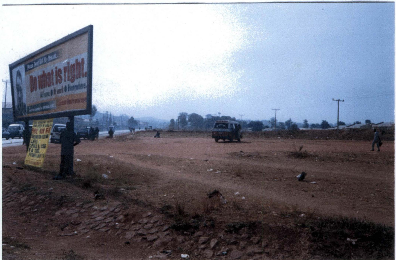
PLATE 6: A typical road lacking avenue planting, in Garki II.
