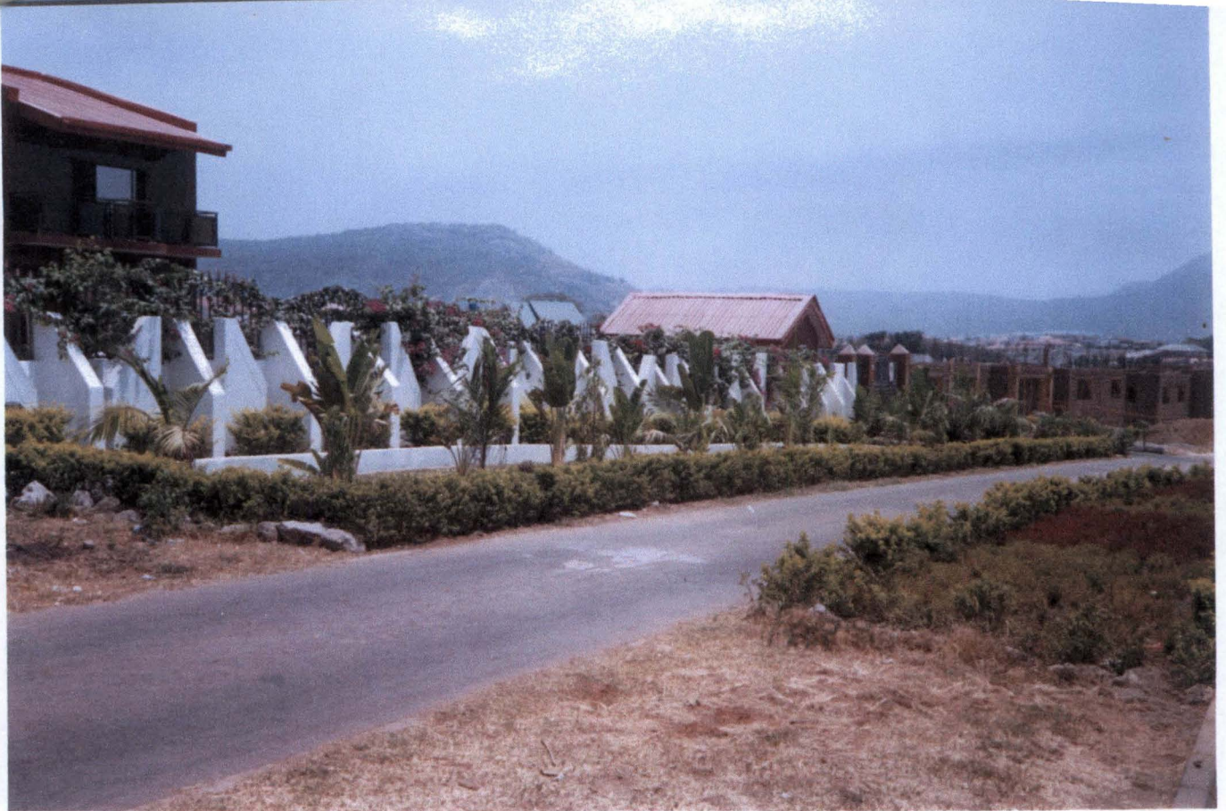
PLATE 7: A Private landscaped house in Maitama district
