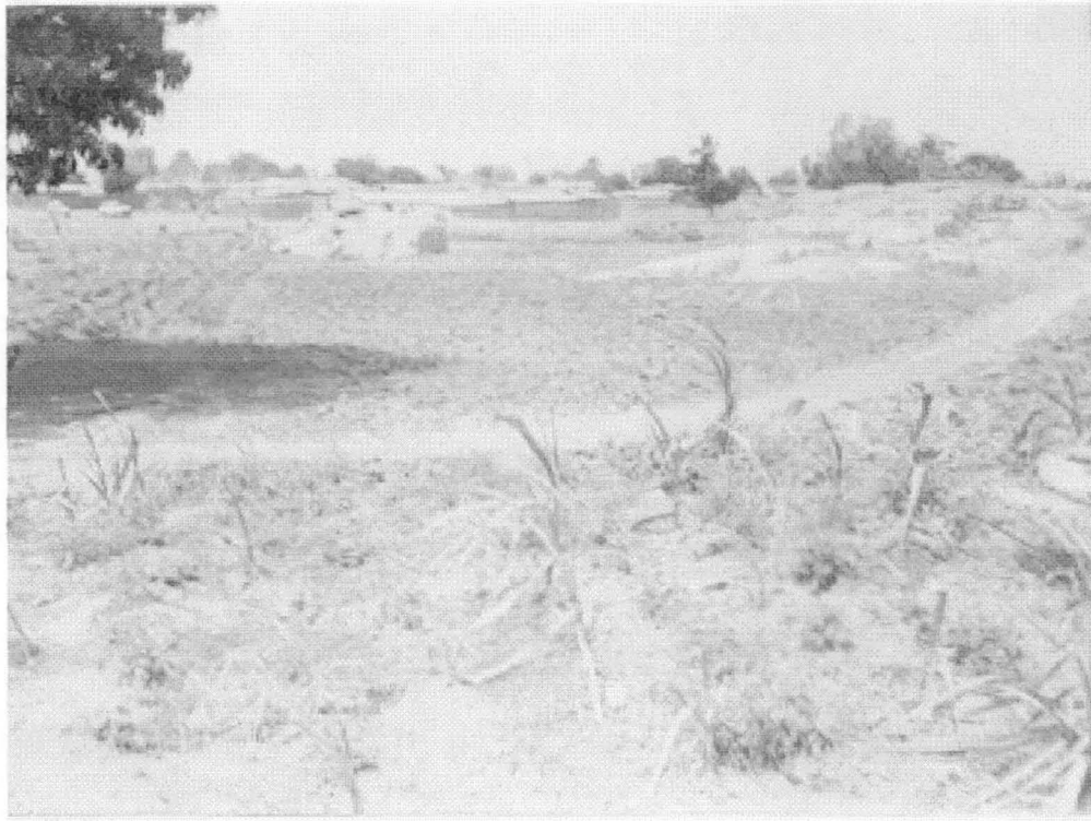
PLATE 9(a): This is the front view of the dam during dry season where it has been tilled for vegetable and sugar cone cultivation..
