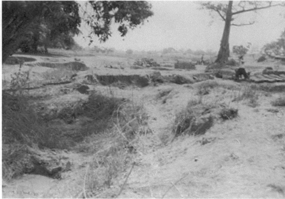
PLATE 6(a): Excavation work for mulding local blocks use in building houses
