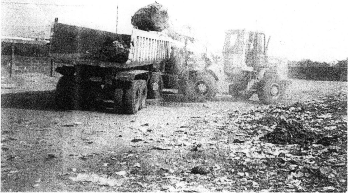
EVACUATION OF REFUSE WITH THE AID OF HEAVY PLANT MACHINES
