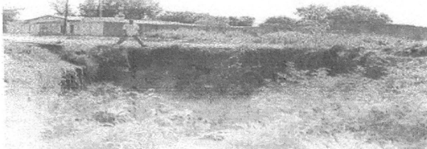
4.2.4: This is as a result of the above poor construction of drainage which led to making this area susceptible to erosion and the menace of land degradation. This is the consequences of lack of E.I.A. (I.s. environment impact assessment).
