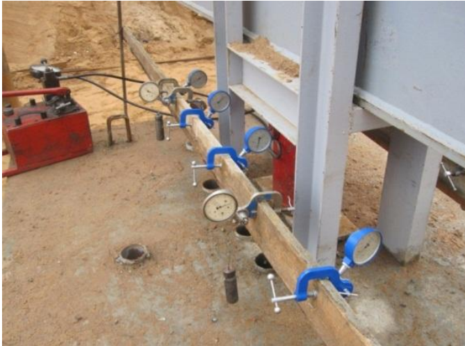
Figure 5. Arrangement of settlement gauges.
