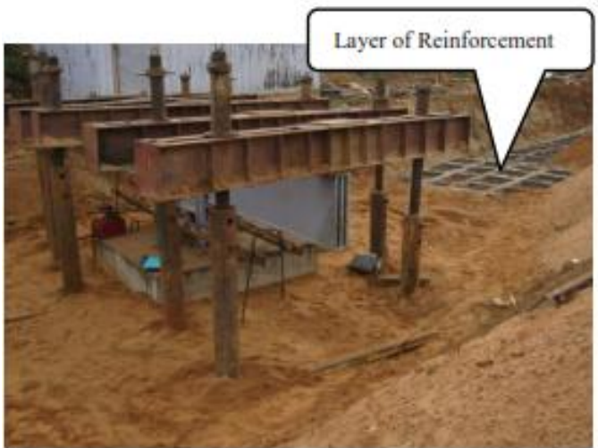
Figure 6. The test set up.
