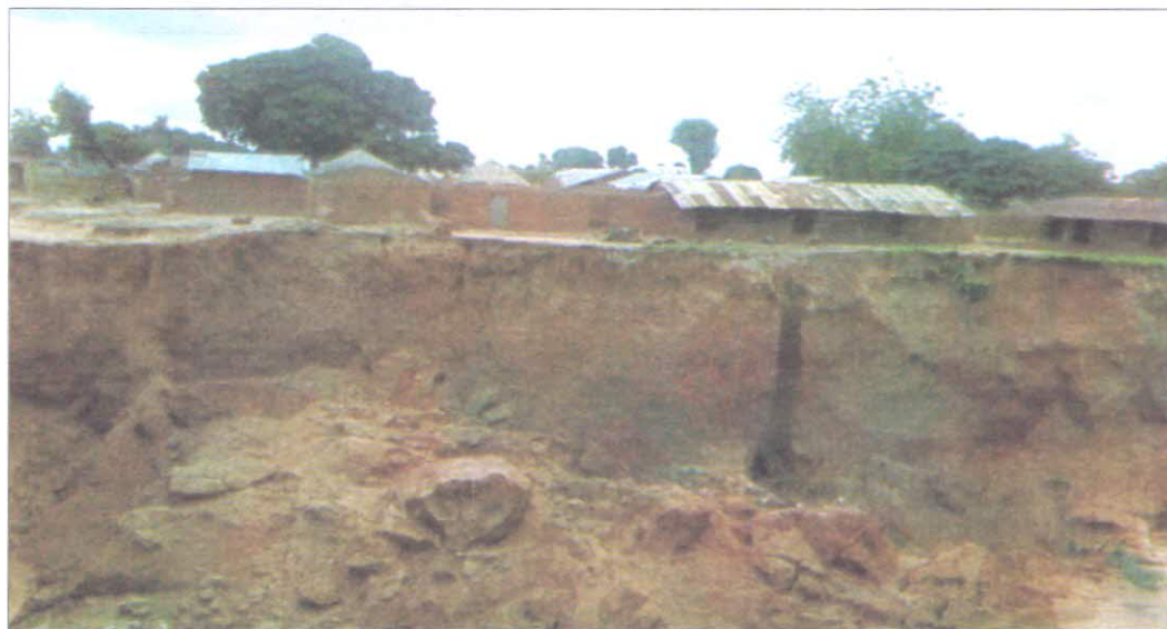
Figure 4. Parts of those houses that are more vulnerable to severe gully erosion.
