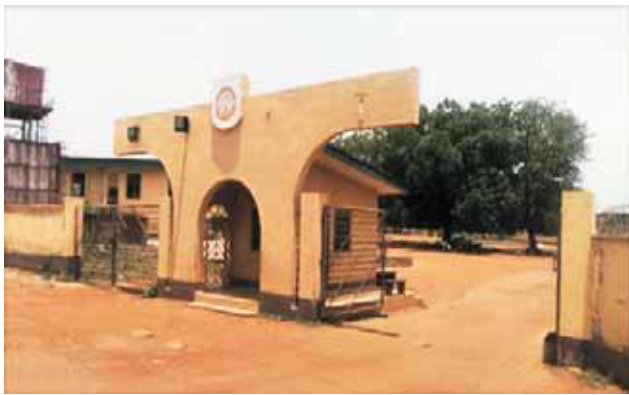
Figure-8: Entrance into the School Environment.
