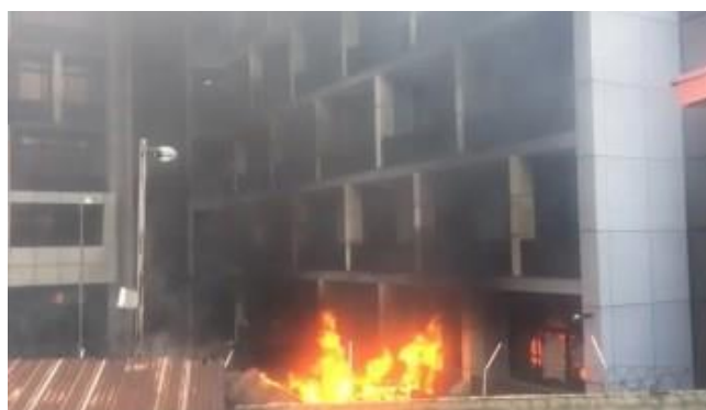
Figure 6: Burning of the NPA building in Marina (Akinrefon, 2020)
