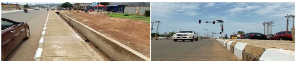
Figure 7. Good transport infrastructure and road furniture in Minna.
