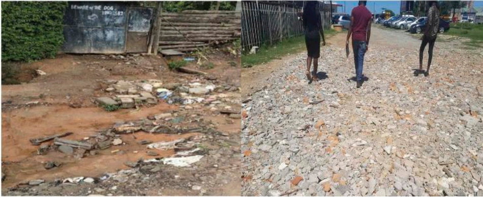
Figure 6. Construction Debris used as filling on roads in Buchi and Nkana West, respectively. Source: Authors
