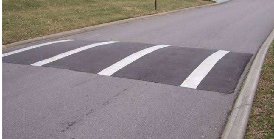
Plate I: Typical picture of a Speed Hump (Source: National Association of City Transportation Officials, 2021)
