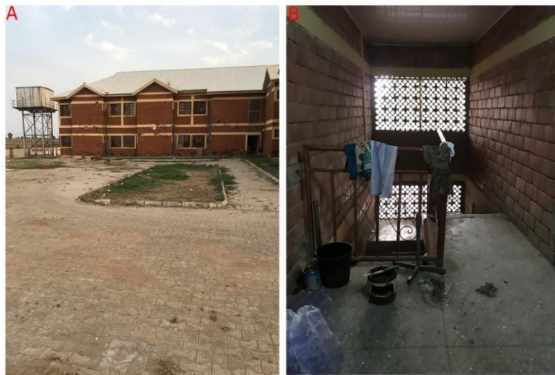
Plate VI: A. The paved area devoid of trees. B. The use of the corridors for cooking activities
