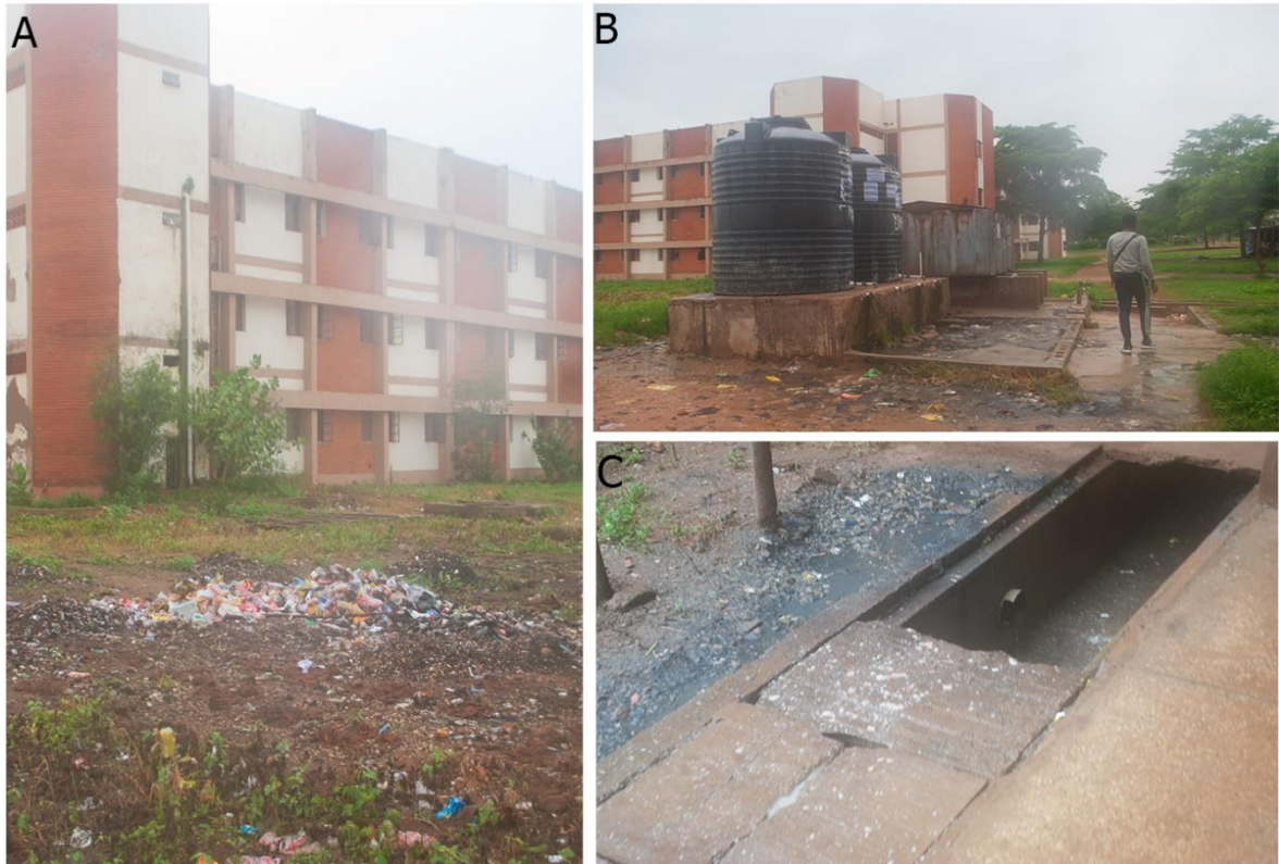
Plate III: A & C. The outdoor environment surrounding the hostels. B. Image of the clogged drainage of the central courtyard.
