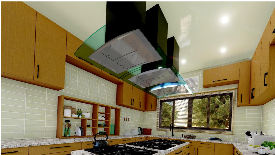
Figure 4.51: The use of extractor fans in the kitchen interior.
