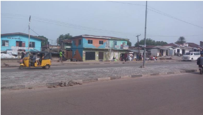
Plate 3: Rehabilitated Road with interlocks (2016)
