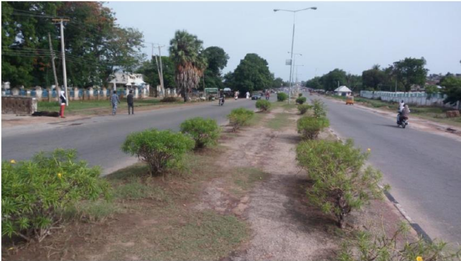
Plate 2: Road before Rehabilitation (2008)
