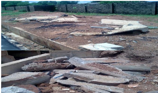
Plate 4: Dutsen kura road concrete waste
