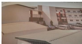
Plate IX: Connection in National Hospital
