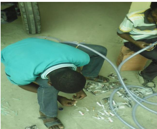
Figure 2a: Fitting of the emitters
