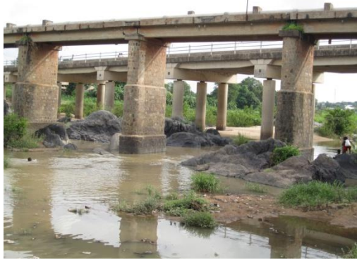
Figure 2: Chanchaga bridge, Minna-Nigeria
