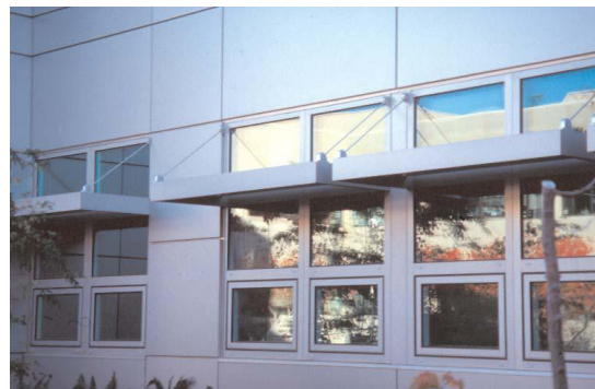
Fig. 5 Light shelves for optimal daylight absorption
