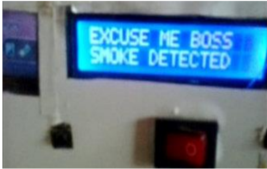
Figure 7: implemented system showing smoke detected
