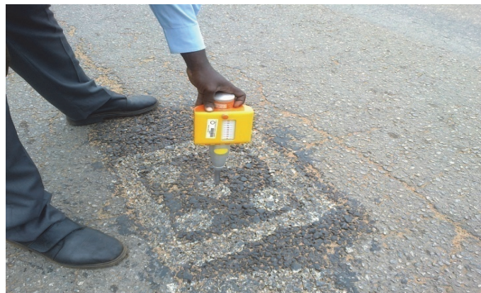
Figure 3: Rebound hammer test
