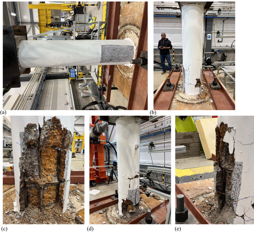
Fig. 15. Observed damage during the cyclic test of Column B1: (a) concrete cover crushing/spalling at 0.8% drift; (b) fracture of vertical bar and severe cover spalling at 2% drift; (c) visible buckling at 3% drift; (d) severe core concrete crushing at 3.5% drift; and (e) hoop fracture at 4% drift.
