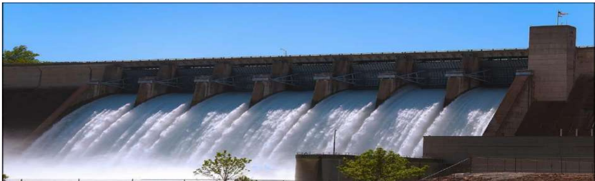
Figure 1 A well-maintained Dam at Zungeru. (Africa Energy Portal, 2020)
