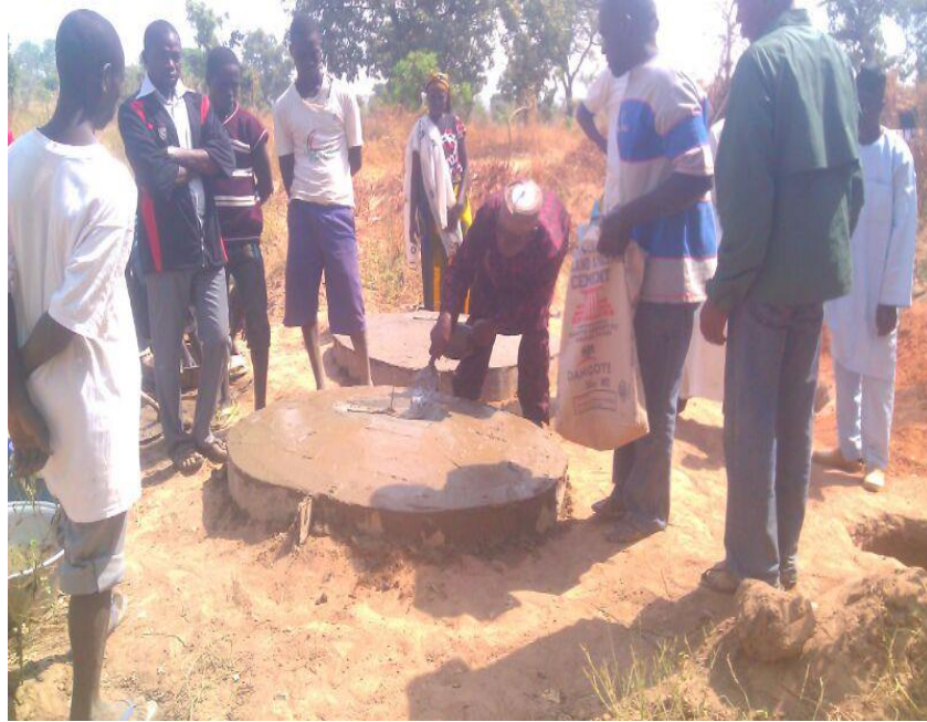
Plate 3. Preparing sanitary platforms for toilets
