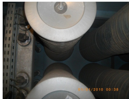
Figure 1. Pulse filters before cleaning
