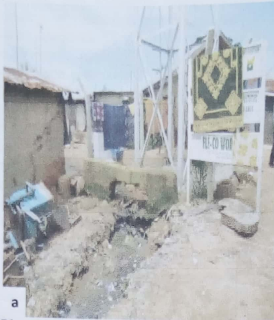
Plate 2(a&b): Discharge of leachate from unlined pit-latrine to the land surface in the study area.
