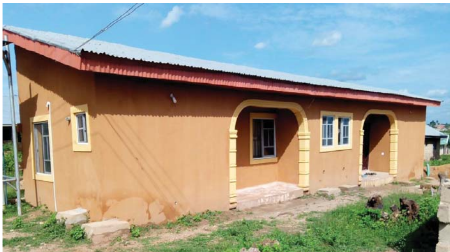
Fig 4: A Room and Parlour Self-contained (semi-detached)
