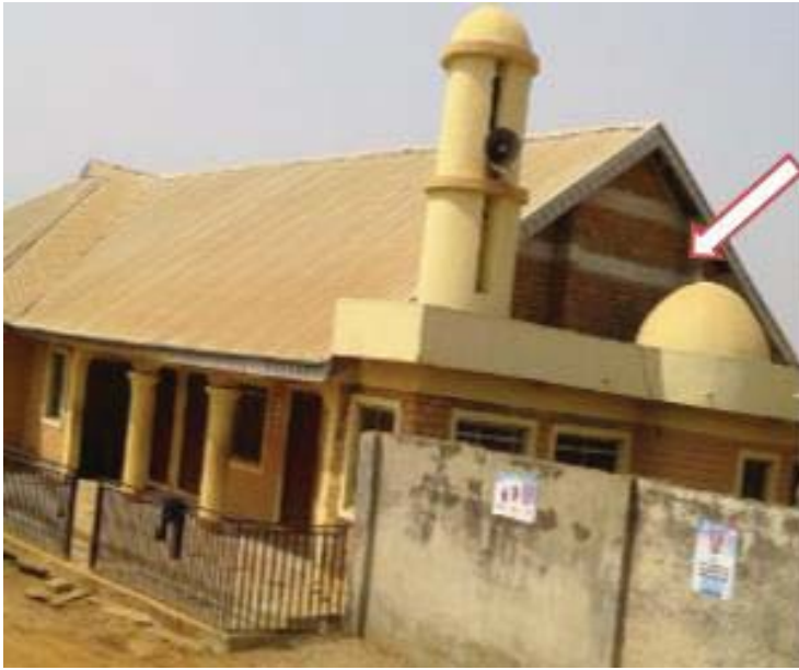
B.1(a): The gable end shown with a pointer collapsed and re-built by introducing vertical pier in the walls
