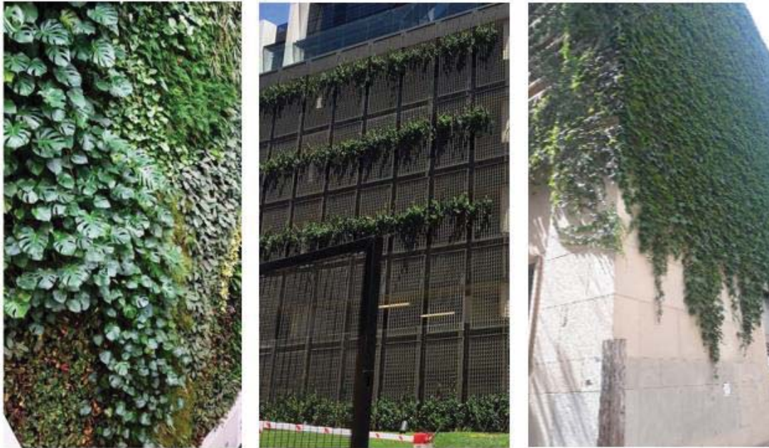
Fig 2: Photo of a living wall indoors (left), indirect green façade (middle) and direct green façade (right)
