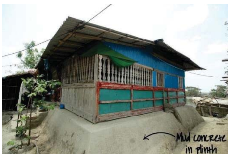
Plate 4: A house in Bangladesh situated on an elevated 'compacted earth' plinth S.B. Linkon, [2017].
