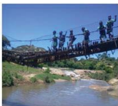
Figure 10: Grade Zero students crossing the dangerous footbridge
