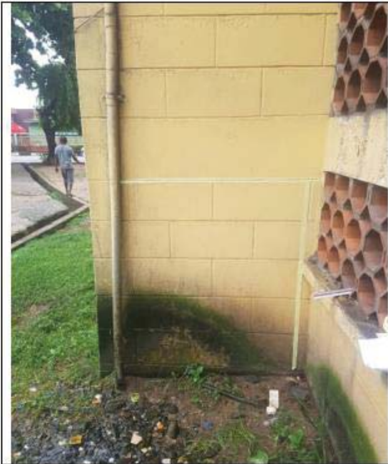
Plate A: The grids being marked out on the wall
